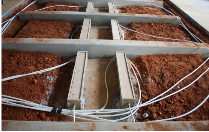
Good installation of the spray nozzles for flushing trench drains.
