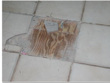
Tile over plywood substrate
