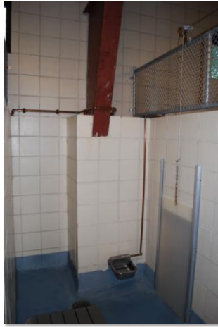
Watering system installed after construction.
