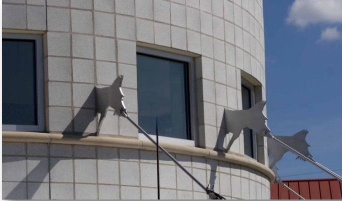
Dog head bracket supports entrance canopy. (Montgomery County Animal Resource Center)
